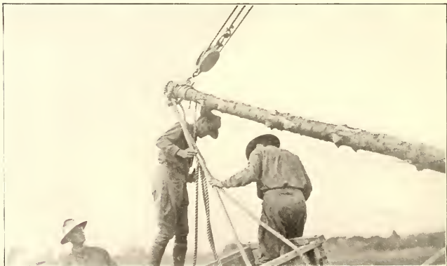
DERRICK AS CONSTRUCTED BY THE M. I. T. CORPS OF ENGINEERS
